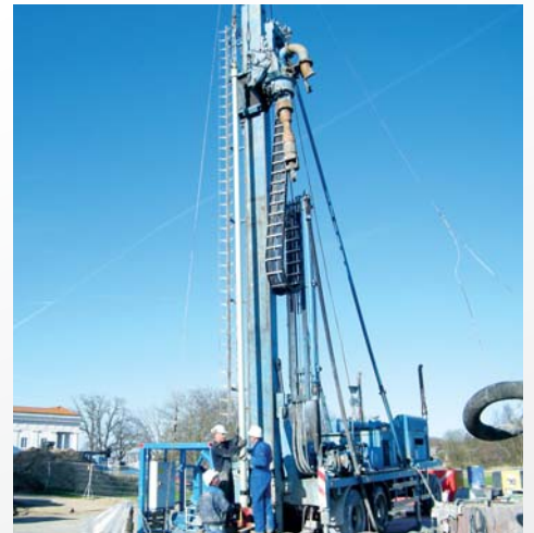
Thermal water drilling at Rügen/Germany
